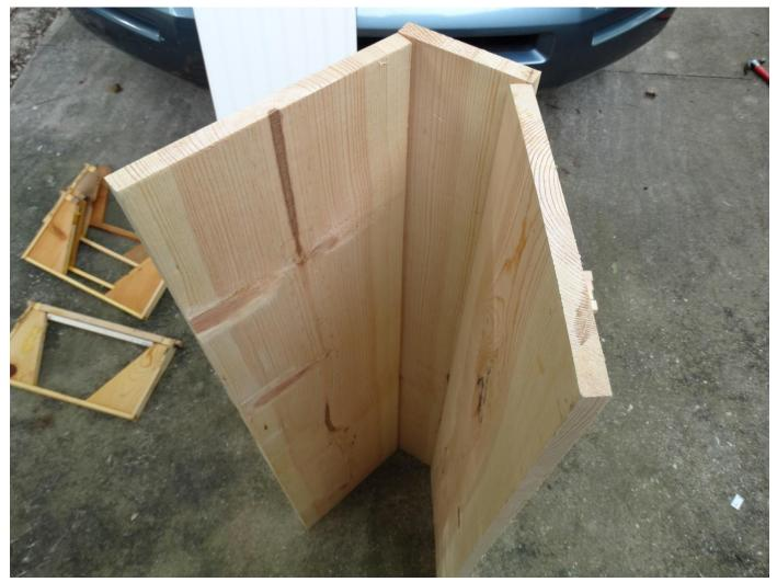
Now spread the sides apart approximately to the extent shown here (some where around 15" for now). Yes, the nails BEND and is why you shouldn't use screws for the bottom attachment. No, you don't need to show off your carpentry skills and calculate bevels... it is fine like shown.
