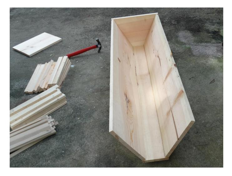
Nail the 15" 1x12 end plates to both ends of the sloped-sided trough. Yes, you may now substituted screws instead of nails. In fact screws are a good idea. Again don't cut anything triangular... just leave the ends straight cut. Remember the goal is quick, cheap, and fast.
